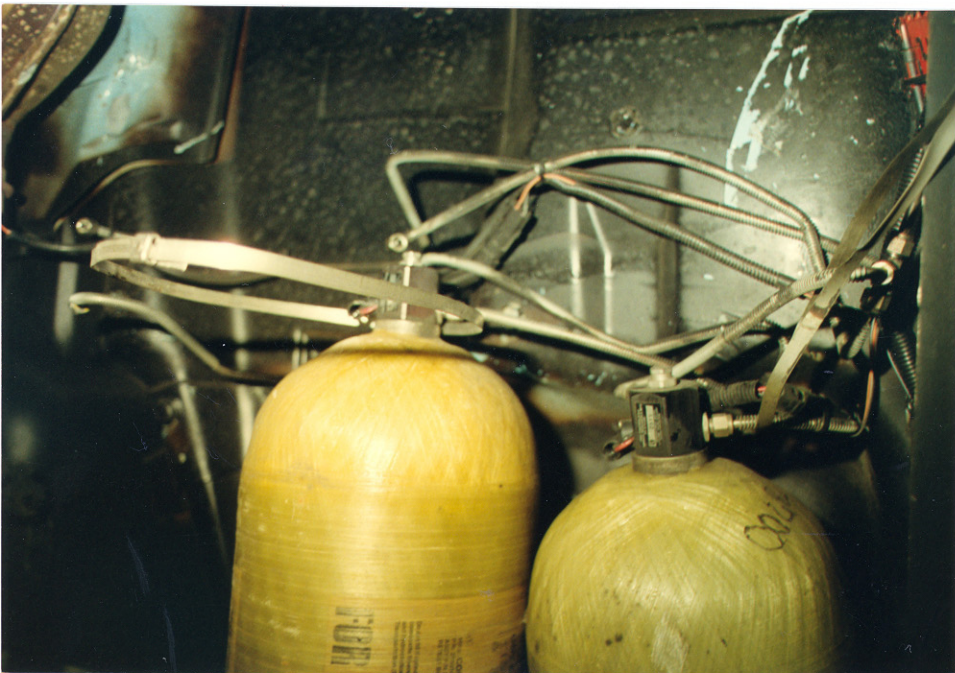
18. Closeup View of the Solenoid Valves and the Armor Tubing
